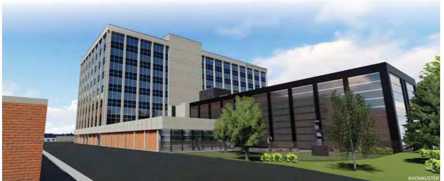
In May, construction will begin on an eight-storey addition on the south side of Barnett House. The project is projected to be complete by the summer of 2018.
